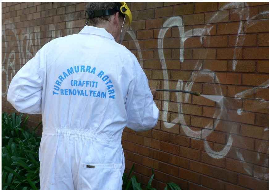
BRICKWORK .....then use water-blaster
