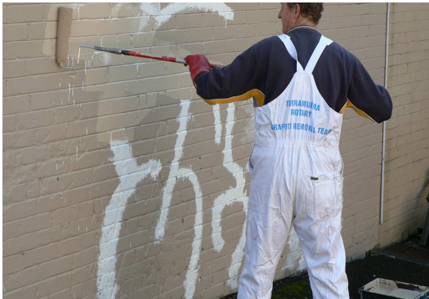
PAINTED SURFACES PrepLock then repaint
