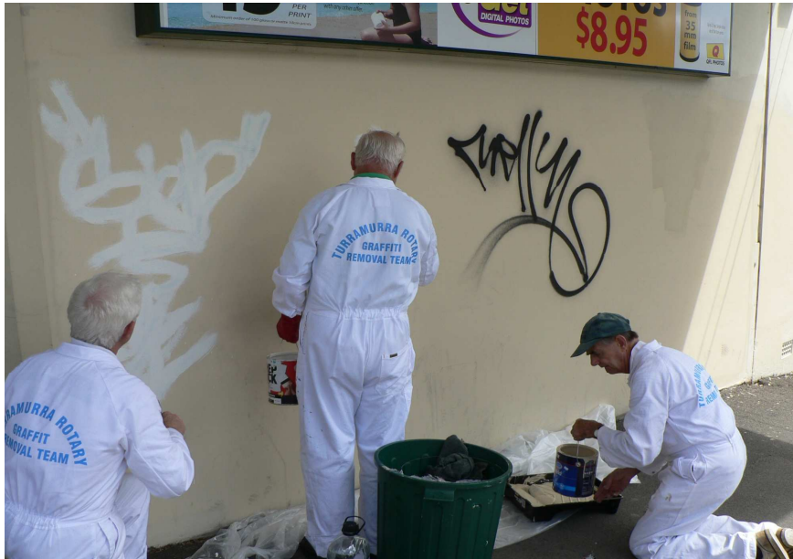
PAINTED SURFACES PrepLock then repaint
